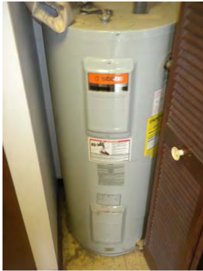
Typical older electric water tank
