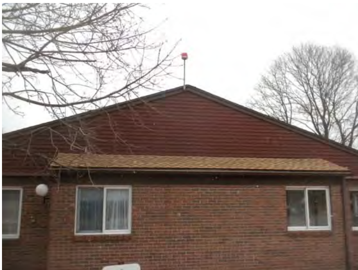
Gable ends are covered with vinyl siding
