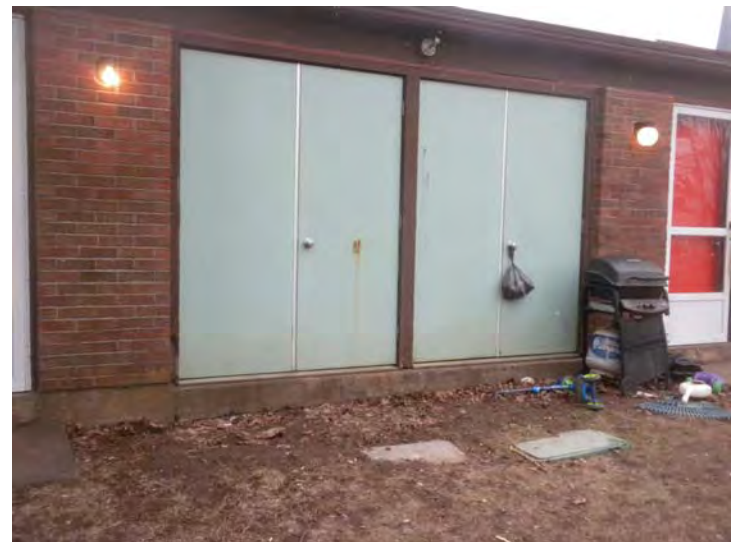
Metal doors to unit electric meters and fire alarm panels
