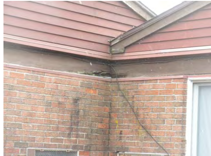
Example of trim wood rot and brick deterioration typical at building corners.
