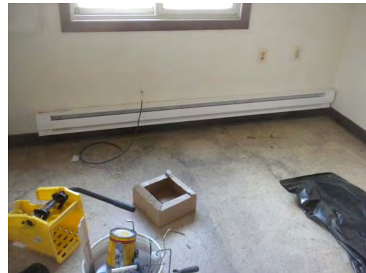
Recently replaced electric baseboard
