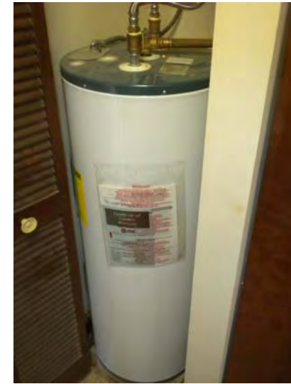
Typical newer domestic hot water tank replacement
