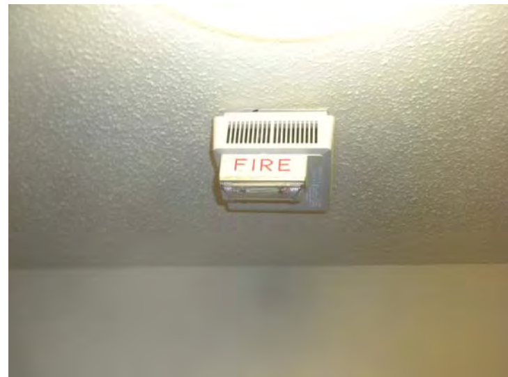
Smoke detectors with horn/strobes report to the fire department
